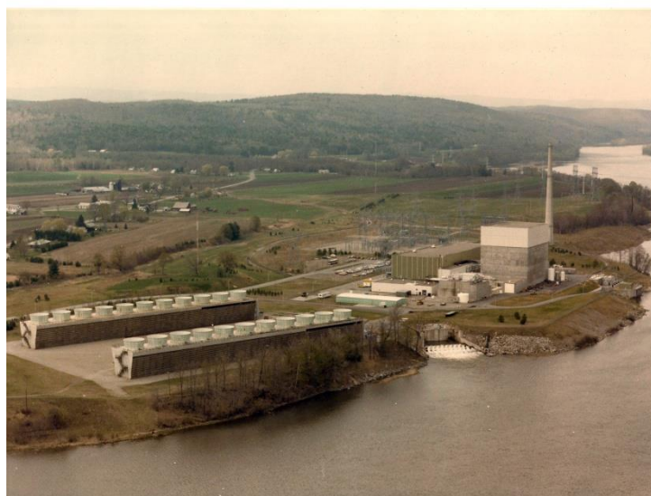
Vermont Yankee. The cylindrical structures in the foreground are the cooling towers, the boxy structure in the middle is the reactor building.
