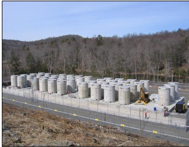
FIGURE 2. 2: SPENT FUEL STORAGE, CONNECTICUT YANKEE
