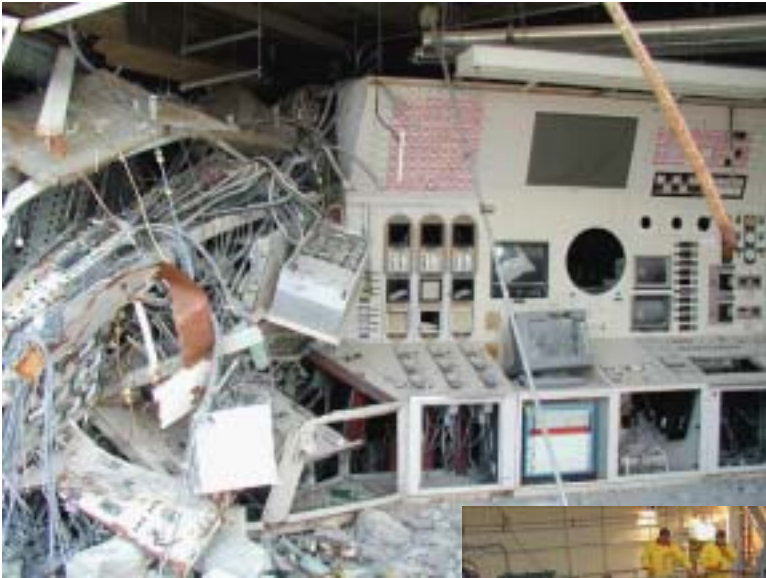
Demolition of the Maine Yankee control room
