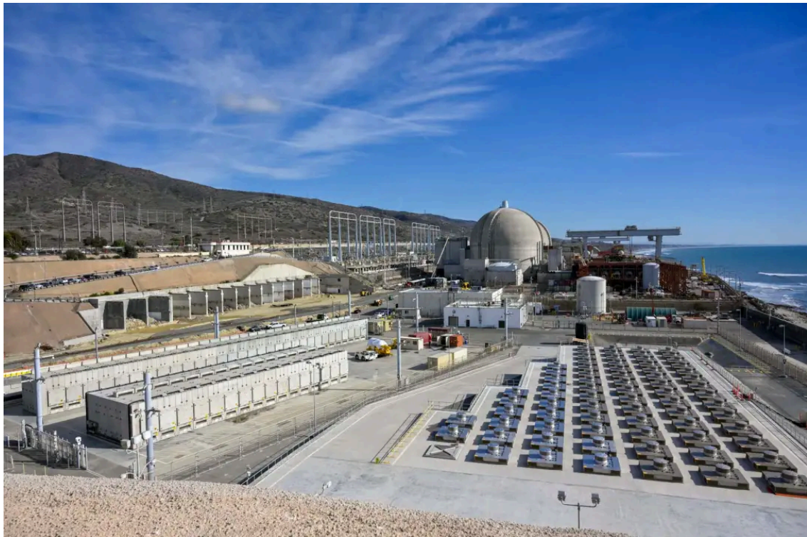
Dry storage of used fuel rods at the San Onofre Nuclear Generating Station in Camp Pendleton, CA, on Thursday, December 16, 2021. (Photo by Jeff Gritchen, Orange County Register/SCNG)
